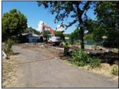
525 Elliott Demolition Work
